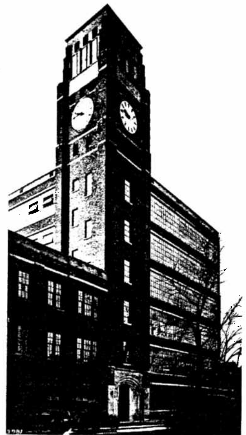
The creativity of Pond & Pond continued throughout its career, as evidenced by this 1926 factory for Bell & Howell, with its then-modern continuous ribbon windows.
